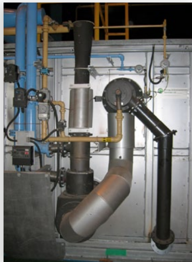
EJ03-07HA connected to a HCR20 Compact Recuperator
